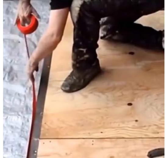
Figure 5 - Installing Red Poly Perimeter tape
