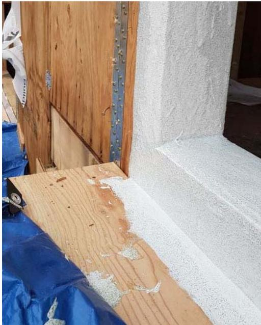
Figure 6 - Waterproofing verticals (door sill)
