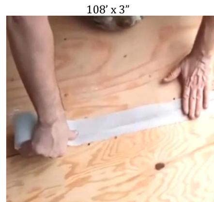
Figure 2: Installing Seam Tape
