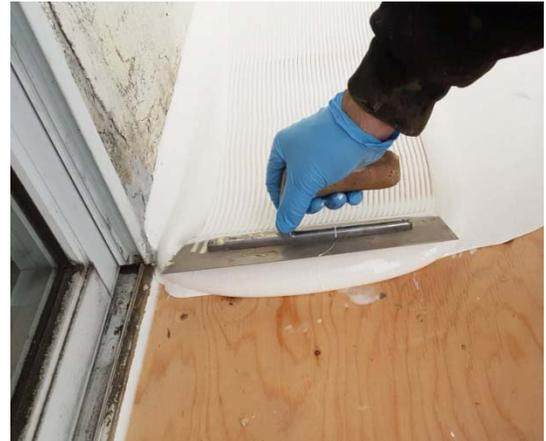
Figure 8: Spreading Base Coat
