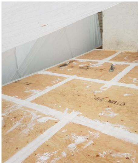
Figure 3: Finished Seam Tape
