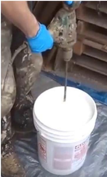
Figure 9: Mixing Base Coat
