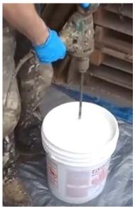
Figure 8: Mixing Base Coat
