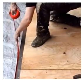
Figure 5 - Installing Red Poly Perimeter tape
