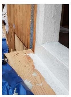
Figure 6 - Waterproofing verticals (door sill)
