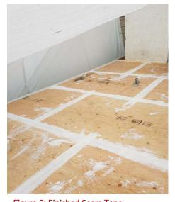
Figure 3: Finished Seam Tape
