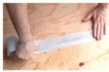
Figure 2: Installing Seam Tape
