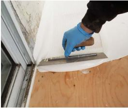
Figure 7: Spreading Base Coat
